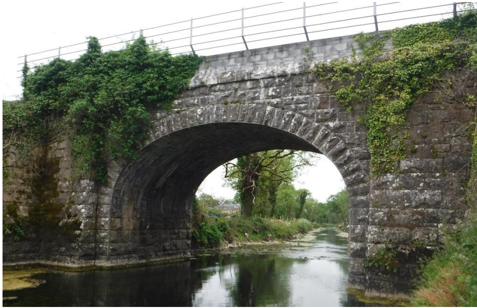
Figure 4; UB154 Railway Bridge
