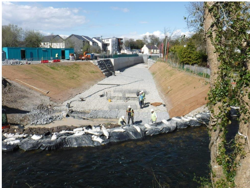
Figure 1; Reno Mattress installation @ Downstream Bypass Channel
